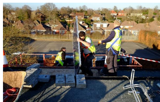
Figure 4 Solar Resources install panels on the Downlands School main building, Feb 2015
